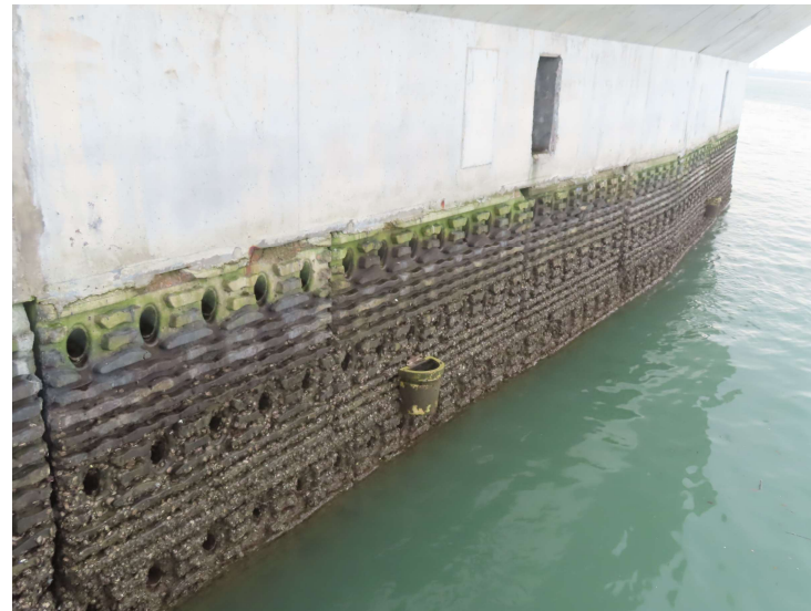
General View of Vertical Eco-shoreline
