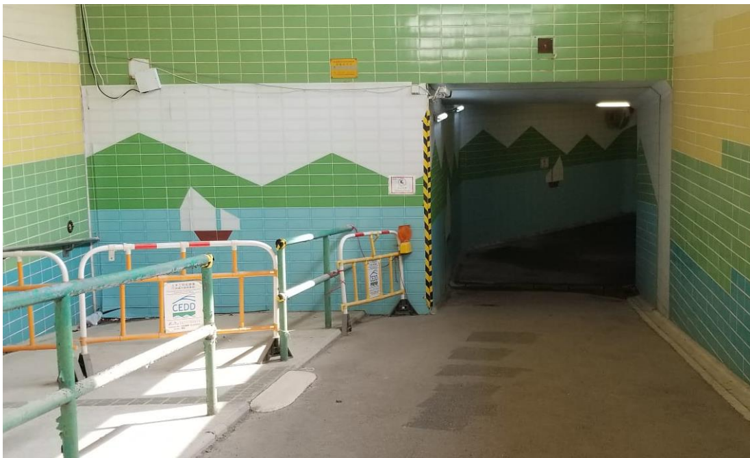
Photo 3 - Erection of site hoardings in unobtrusive colours
